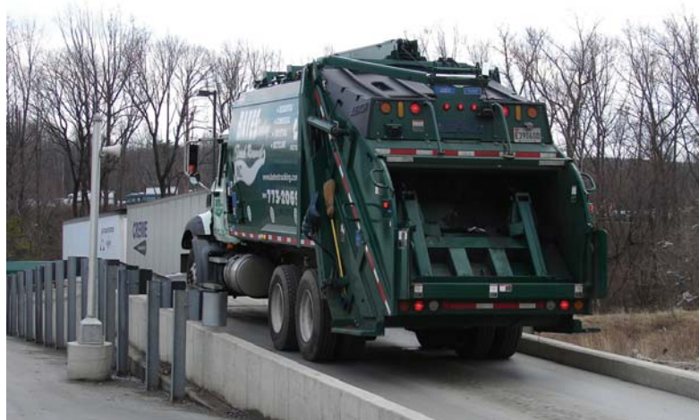
The inbound weighbridge required a ramp 150 feet long to provide a safe incline for trucks delivering recyclable materials.
